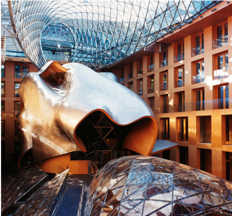
The distinctive office block of DZ BANK, designed by star architect Frank O. Gehry, accommodates DDV's Berlin office.
